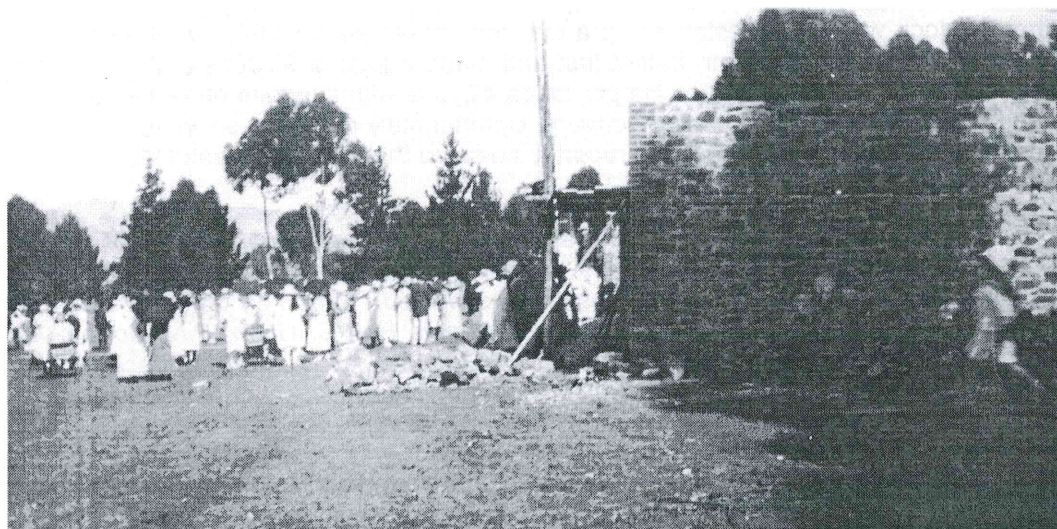
The pavilion under construction
